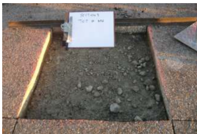
Figure 3.6. Two foot by two foot test area after asphalt removal (Section 3).
