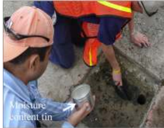
Figure 3.18. Subgrade moisture content sample.
