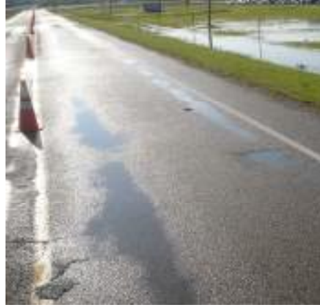
Figure 4.37. Ponding in six-inch thick sections in May, 2011 (from Goldman, 2011) [view from Section 13W looking East].
